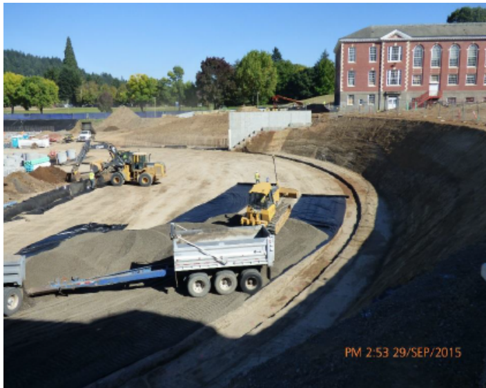
Gravel installation for the Cement Treatment Zone South End of Field
