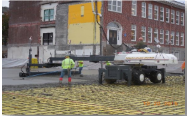
Slab On Grade Placement with Laser Screed
