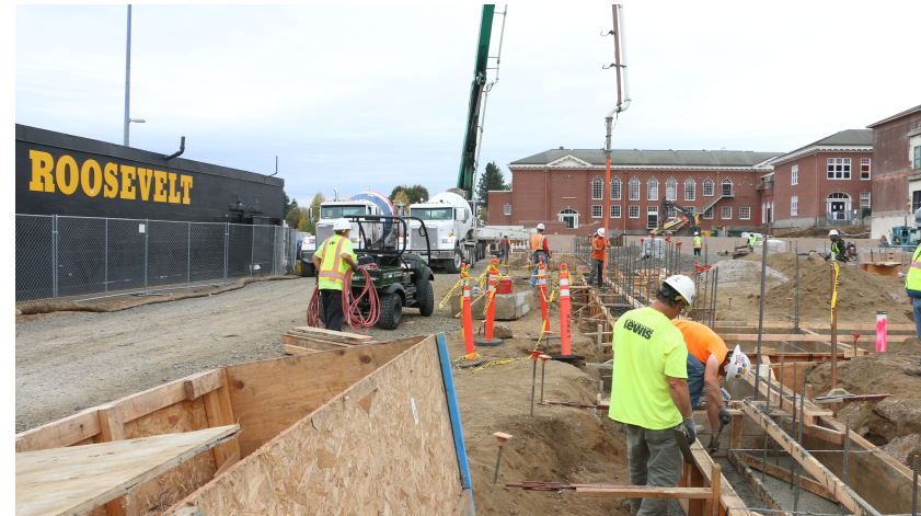
New Gym Footings
