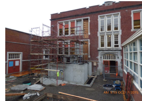
Ainsworth Elevator Shaft
