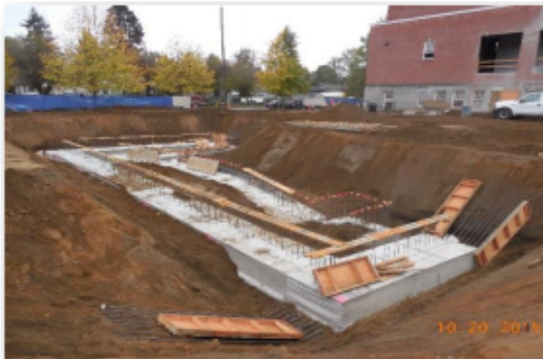
Orchestra Pit Continuous Footing Placed with Backfill Ongoing
