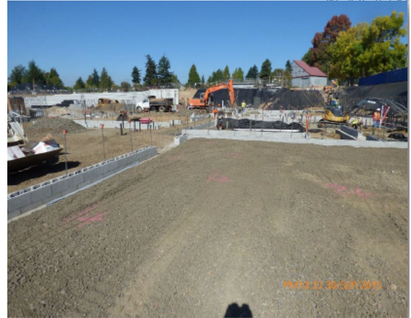
Sector 7 Building Pad Placement (Rm. 7018 Exercise/Wrestling)
