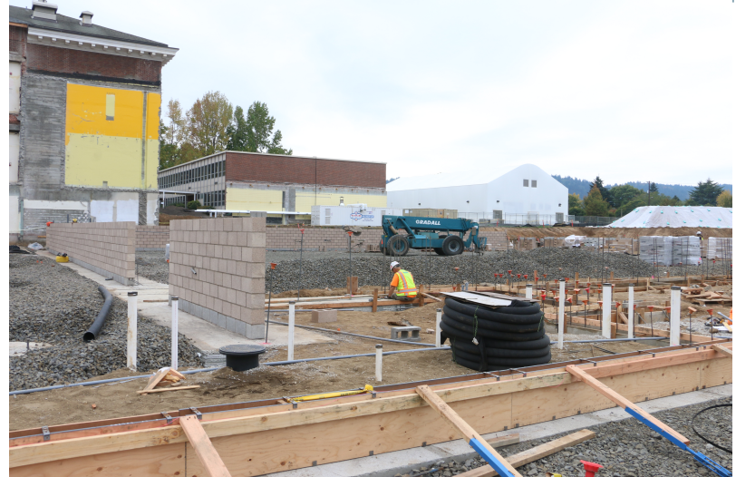
CMU Walls for Gym (Area C)
