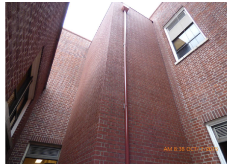
Woodlawn Elevator Shaft
