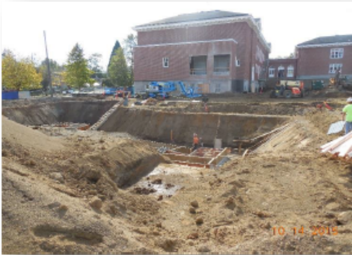
Orchestra Pit Continuous Footing Formwork in Progress
